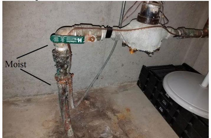
This is a typical water meter located in a residential basement. Although difficult to see here, the pipe to the left, located below the meter shut-off valve (the green lever) is moist and shows indications of a leak.
